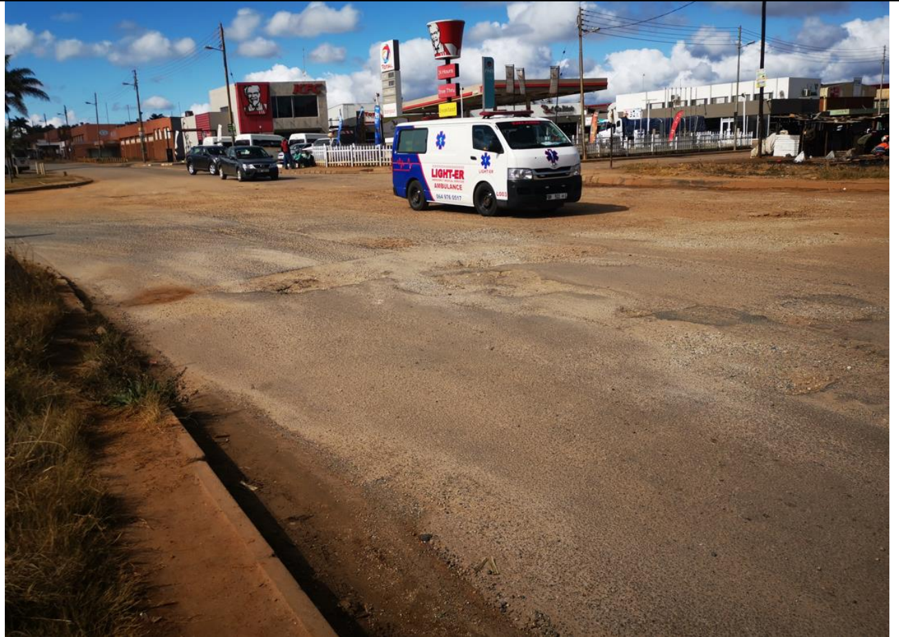
Damaged concrete slab intersection
